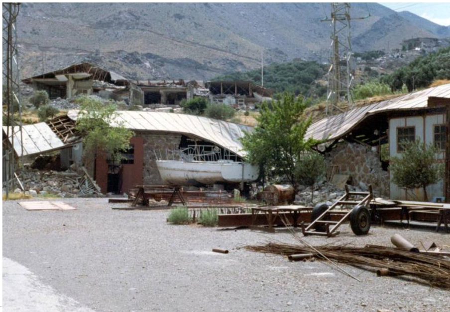
Collapsed buildings at Sefid Rud dam site
