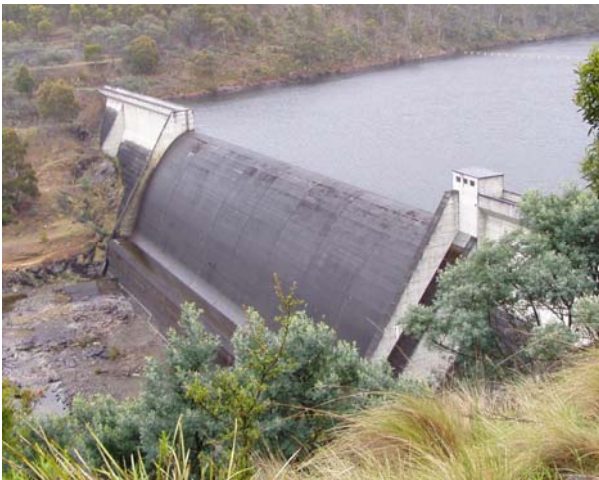
Figure 1 – Catagunya Dam Prior to the Dam Restoration Project Works
