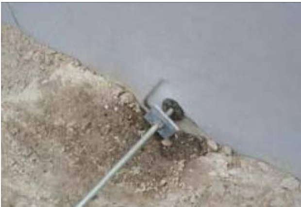
Figure 8. Detail of anchoring rod.
