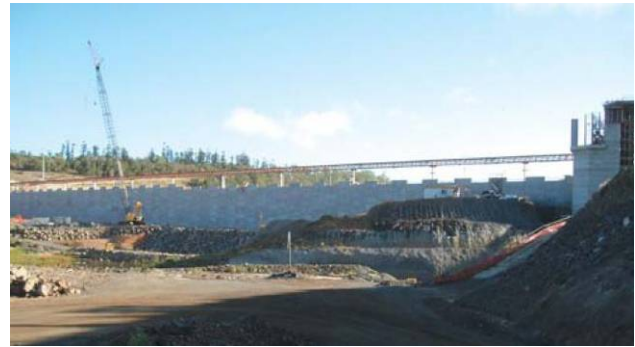
Figure 10. View of the upstream face as construction works proceeded.
