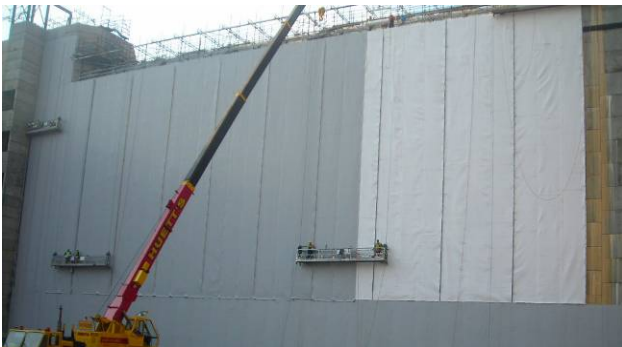
Figure 18. Installation of the PVC sheets (the grey material) on the anti-puncture geotextile in the lower part of the dam.
