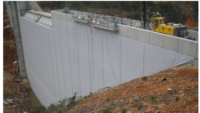
Figure 20. View of the completed geomembrane system installation.
