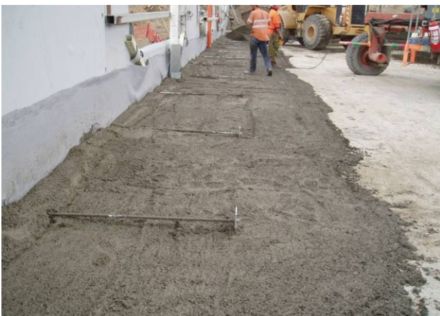
Figure 9. View on the inside face of the panels, showing the steel bars anchoring the panels to the dam body.
