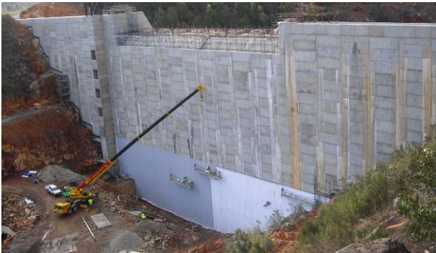
Figure 18. Installation of the PVC sheets (the grey material) on the anti-puncture geotextile in the lower part of the dam.
