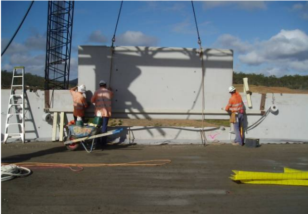
Figure 7. Erection of precast panels.
