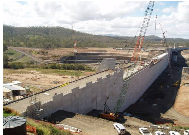
Figure 3. View Paradise Dam from the upstream side during construction in 2005.
