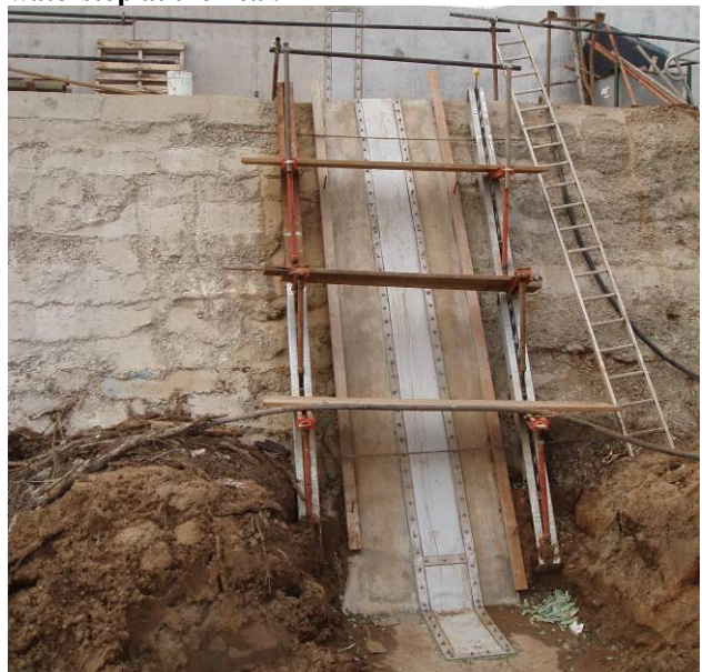
Figure 27. Arrangement of the connection to the waterstop at the heel.
