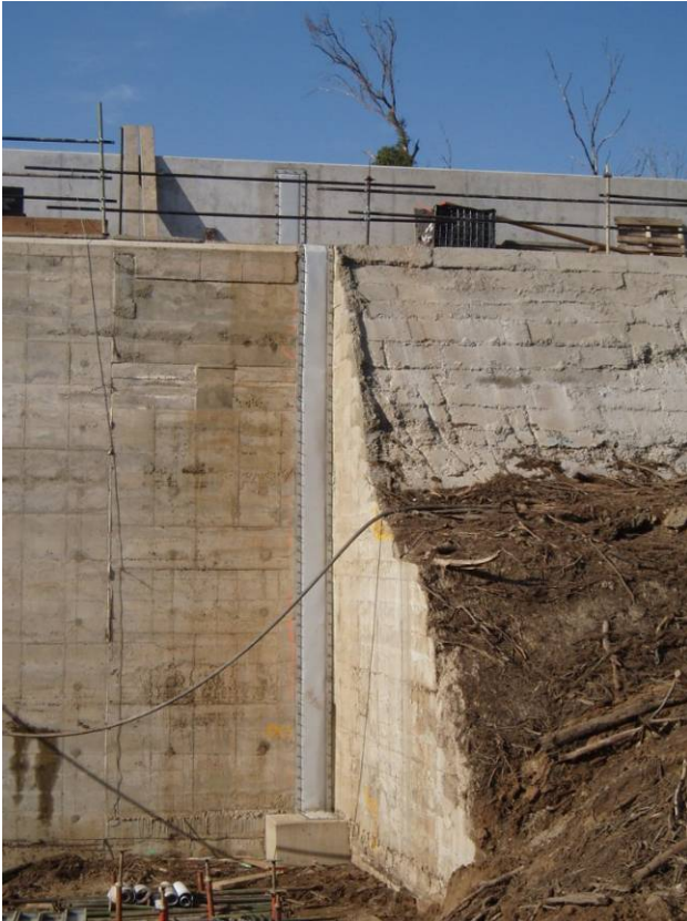
Figure 29. View of the corner waterstop.
