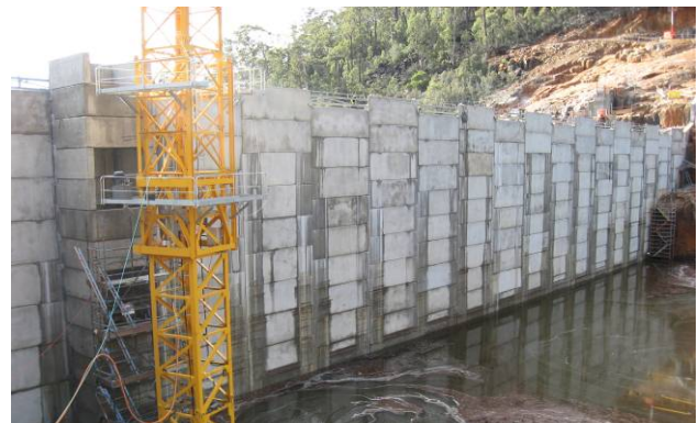
Figure 9. View on the inside face of the panels, showing the steel bars anchoring the panels to the dam body.
